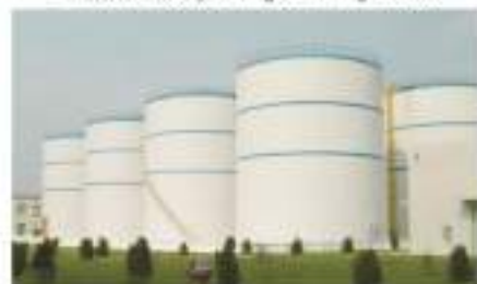
精炼油罐区 Refined Oil Tank Area
