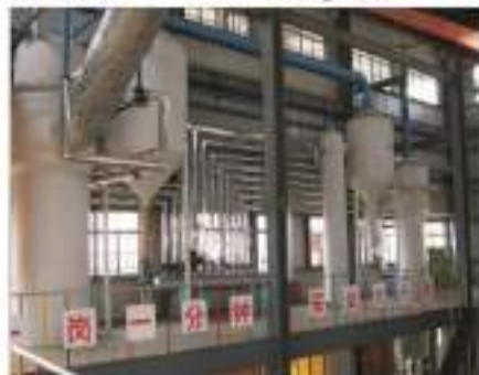
浸出车间上部 Upper Part of Extraction Workshop
